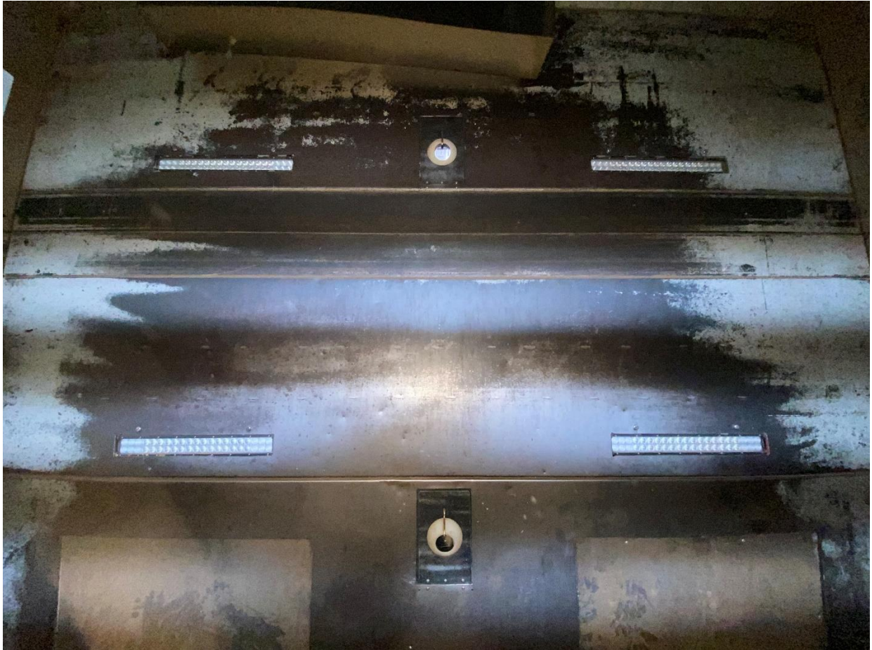
Figure 5a. Interior photo of module feeder inspection system cameras and lights installed on the back wall of a module feeder.
